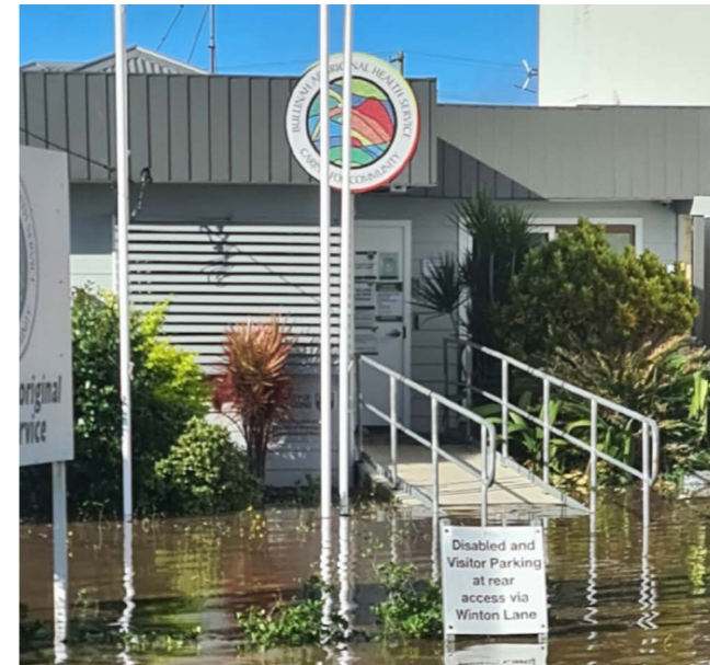
Main Clinic front entrance
